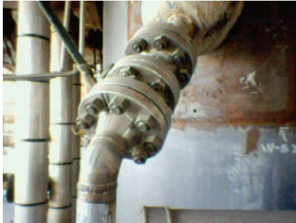
This CA-DRI 2-inch ASME 300 class isolation valve handles the withdrawal of hot spent catalyst from the regenerator.
