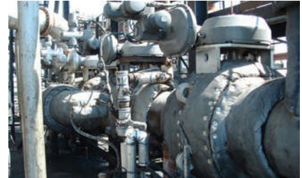
This midwestern refinery has four 20-inch ASME 300 class MOGAS ball valves in overhead vapor service. Several are beginning their second decade of service.
