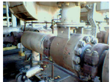
This clamped end CA-HO1 10-inch ASME 2500 class catalyst valve installed in 1995 is still in service at a major Italian refinery.
